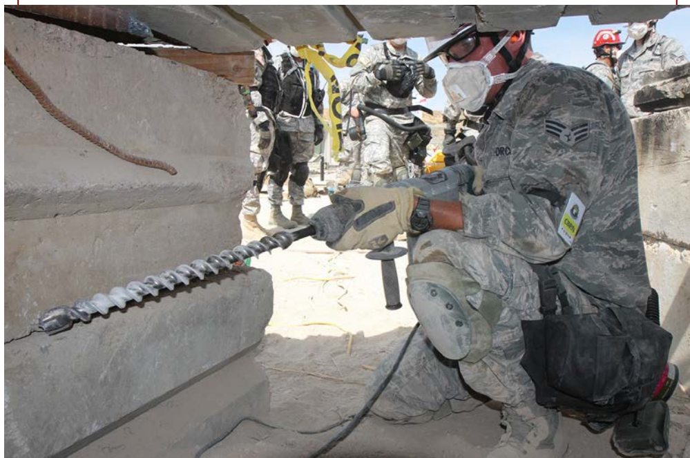
U.S. Air Force Senior Airman Chris Dugger, a firefighter with the 152nd Airlift Wing, Nevada Air National Guard, uses a hammer drill to bore through the concrete wall of a rubble pile to test the air quality behind the wall during Vigilant Guard 2013 in Northglenn, Colo., July 24, 2013. Vigilant Guard is a series of federally funded disaster-response drills conducted by National Guard units working with federal, state and local emergency management agencies and first responders. (DoD photo by Spc. Zach Sheely, U.S. Army National Guard/Released)
